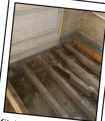
Kitchen Floor Bearers Before Repair Work
